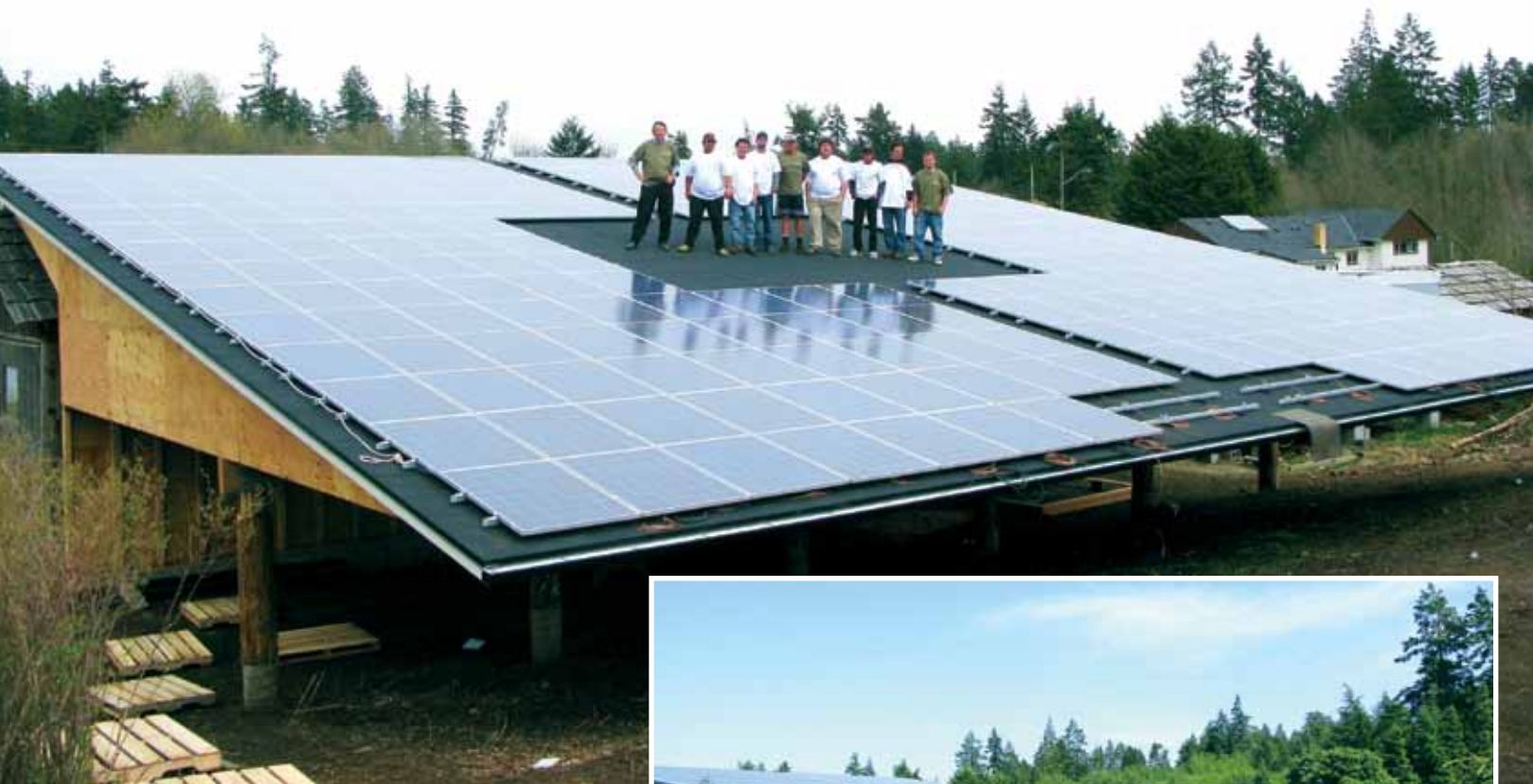
T'Sou-ke Trainees completing 40kW Photovoltaic System.
